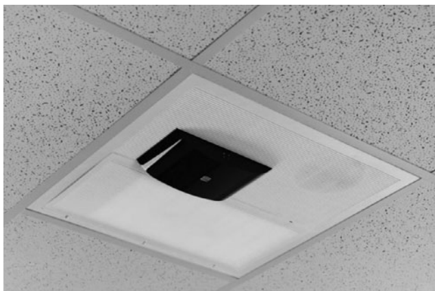
FIGURE 37.9 Classroom audio distribution system placed in the ceiling. [Photo courtesy of Lightspeed Technologies, Tualatin, OR.]
